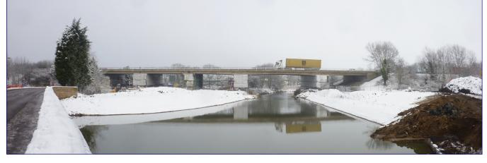
Having been at the centre of local media attention, the A14 River Ouse Viaduct was considered a risk to public safety due to unpredictable spalling of concrete from various sections, in particular were those sections spanning the B1044 road & its walkways. In addition to this the viaduct had generally become deteriorated & required maintenance in order to ensure its ongoing safe use for the millions of users & their vehicles that drive over it every year.
